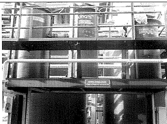
HTDS Treatment Skid Flash Mixer – Coagulation & Flocculation System & Lamella Clarifier
