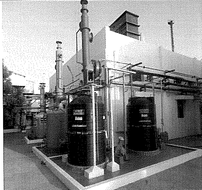
Final Treated Water Collection Tank for Recycling
