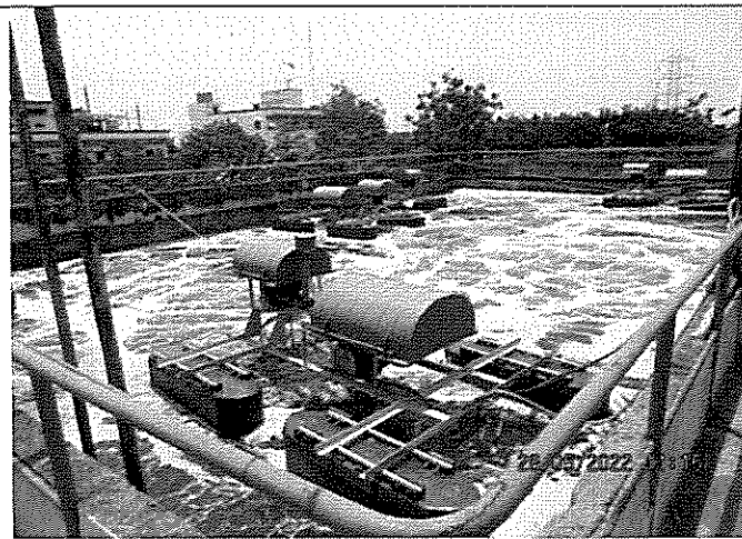
Aeration Tank-02 & Jet Aerator
