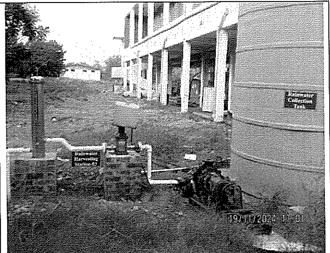
Rain Water Harvesting Station-02 Capacity: 20 KL FRP Tank (Area Behind QC Block-C)
