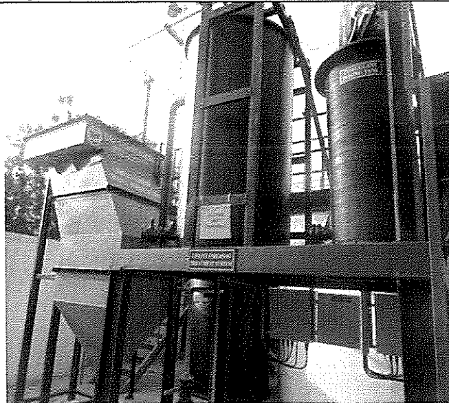
Utility Treatment Skid Flash Mixer – Coagulation & Flocculation System
