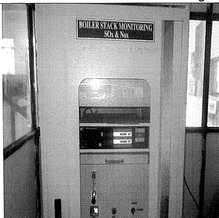
Boiler Stack- Sox & Nox Analyzer
