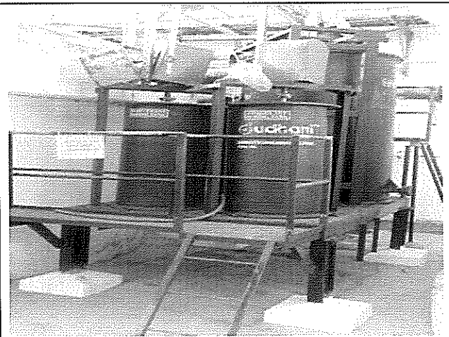
Flash Mixer – Coagulation & Flocculation System
