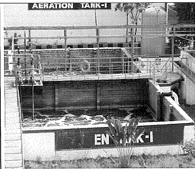
Equalization & Neutralization Tank
