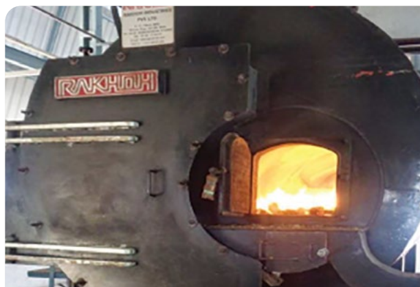
^ Use of Green Fuels (Briquette fired boiler) at NATCO Pharma
